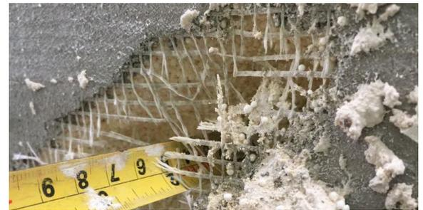
Figure a. Thickness of the isolation layer
